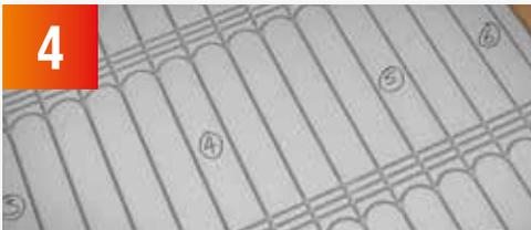
Uplift the numbered boards and prime the underside of the boards with Ultra Floor Prime-IT MSP bonding primer. This should be applied by brush or roller in a thin film. Allow to thoroughly dry to a clear green film ensuring primed face does not come into contact with other boards, walls or subfloor until it is ready to be bedded.
