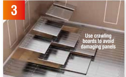
3 Lay the boards across the floor with the grooves facing upwards, making sure the pipework runs are calculated correctly to reach manifold position. Use crawling boards to avoid damaging panels
