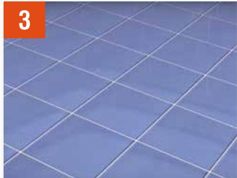
**3** Grout the tiles using UltraTile Flex Joint grout. Allow to fully cure before trafficking.
