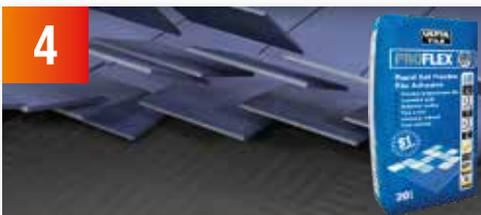
Fix the tiles using UltraTile ProFlex SP adhesive. Ensure full compression of the adhesive to give a void free full adhesive bed. Allow the adhesive to cure for a minimum of 4 hours (depending on temperature) to ensure the adhesive has gone through its initial set before carrying out any further works.
